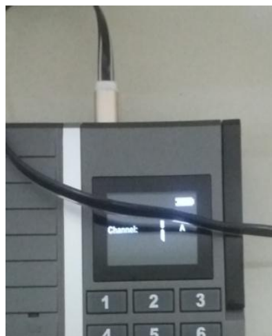
do not put the cable on the surface NG
