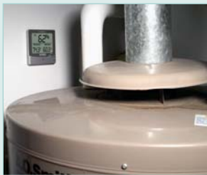
Monitoring Dew Point levels in a Basement for potential mold growth.
