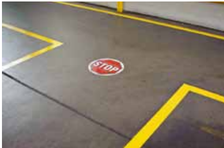
Aisleways & traffic lanes (yellow)
