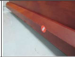
POOR PAINTING ON SPEAKER WINDOW
