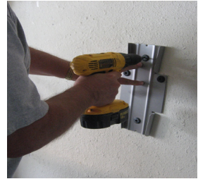
Fig. 2 Mount the wall bracket.
