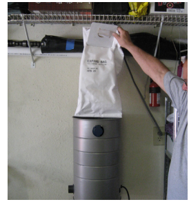
Fig. 1 You will need to be able to remove the bag from the top of the unit. Be sure to leave enough room when mounting.
