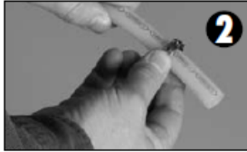
2 Slide clamp or crimp ring over tube.
