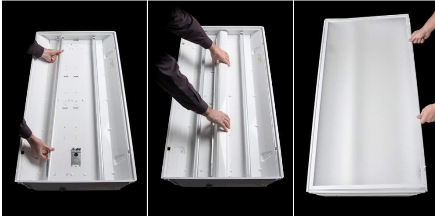
a) Install LED Tube Lamp b) Replace Ballast Cover c) Replace Troffer Lens
