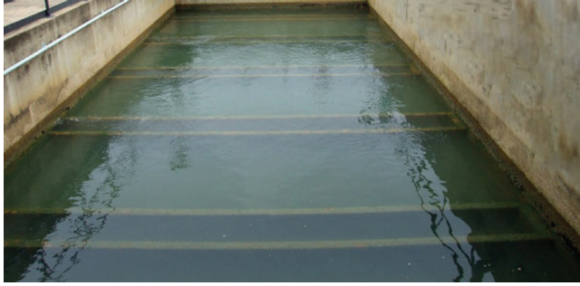
Figure 23.5 Rapid sand filter bed.
